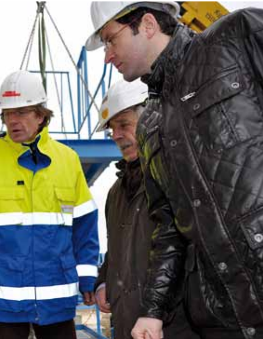
installation of a large number of HEROSE valves
