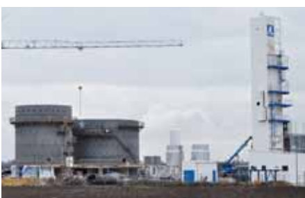
The Gundelfingen construction site in January
