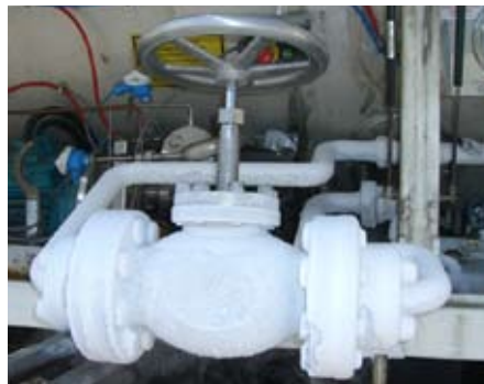
Cold shock testing as per DIN EN 12567 on an LNG trailer (tank truck)
