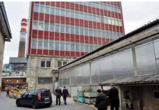
The BMT plant in Brno
